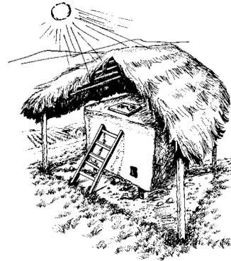
*A well-designed grain store made of bricks or cement*
